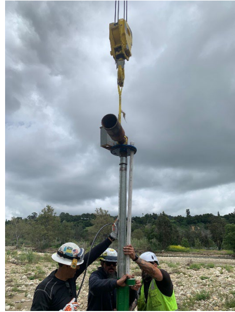
Photo 2. Lowering pump into well. 1.25-inch PVC sounding tube is visible to the right of the pump column.
