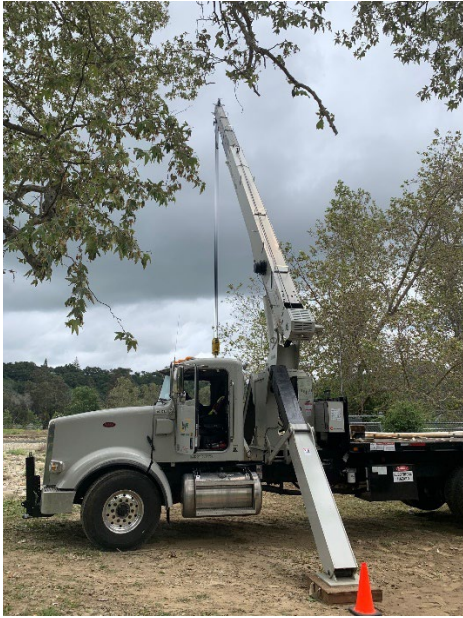
Photo 1. Crane used to remove and reinstall pump.
