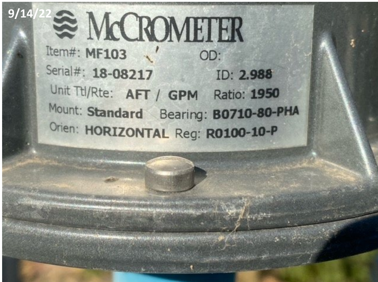
Photo 3. Example photo showing flowmeter serial number for compliance with Well Registration Form Item No. 6(d)(vi)(3).
