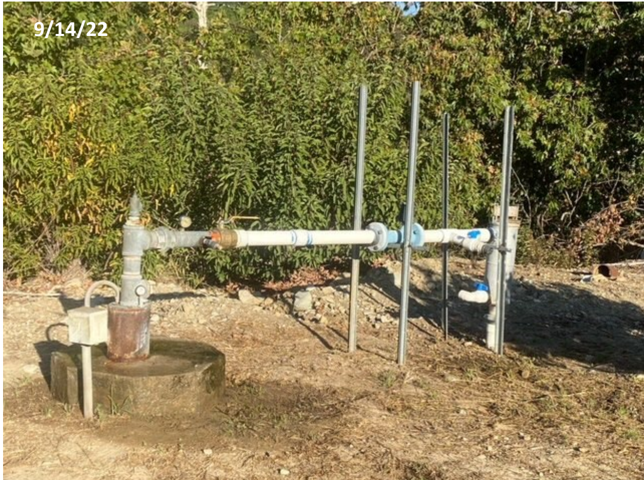
Photo 1. Example photo showing the well and well discharge piping with flowmeter location visible for compliance with Well Registration Form Item Nos. 3(o) and 6(d)(vi)(1).
